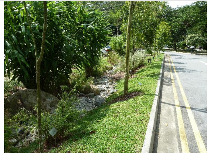
Example 1 of vegetated bioswale
